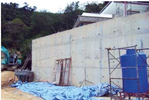
Retaining wall constructed with sufficient drainage.
